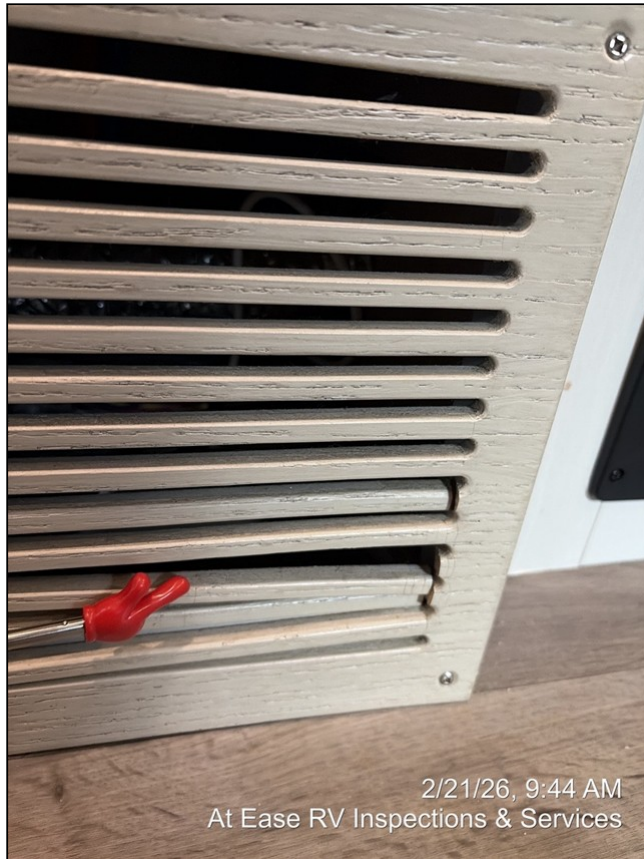
24.24 Item 3 (Picture) Converter/inverter access panel
