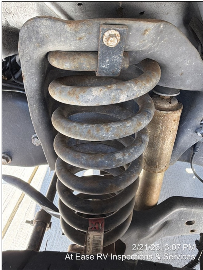
13.5 Item 1 (Picture) Front streetside shock absorber
