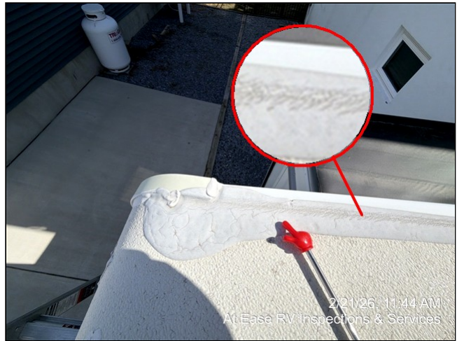
8.3 Item 2 (Picture) Rear wall sealant
