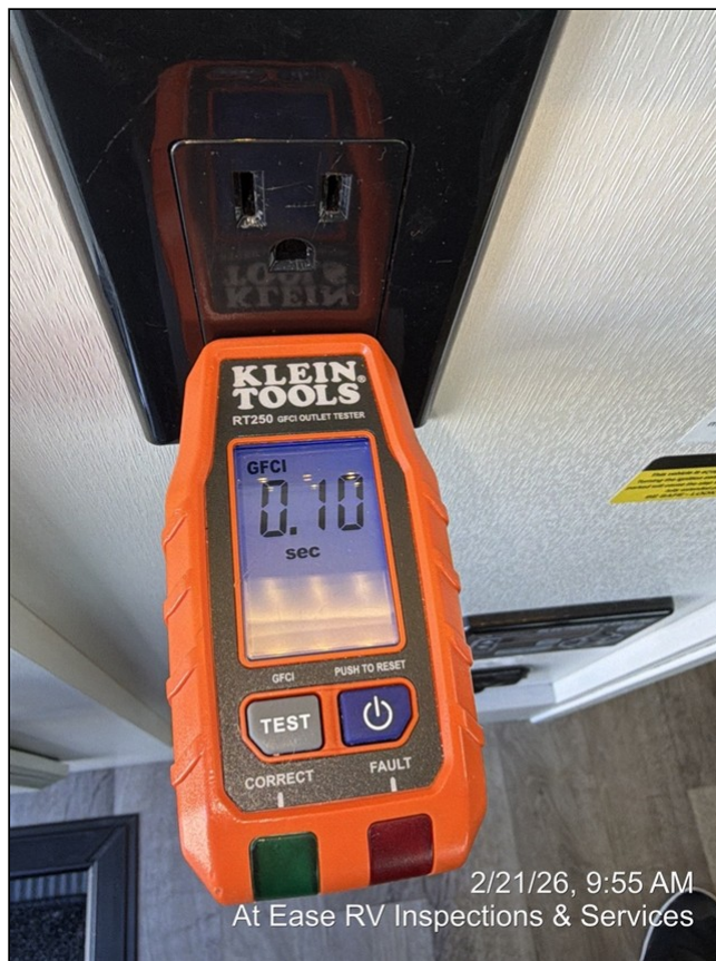
18.13 Item 1 (Picture) GFCI testing
