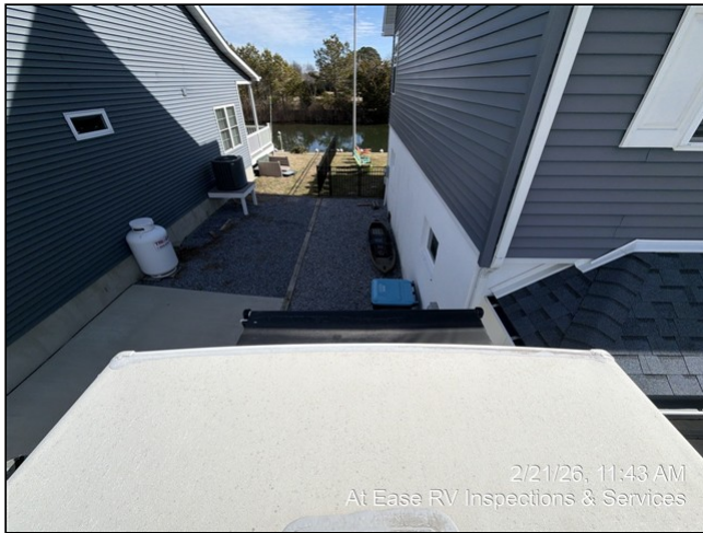
8.3 Item 1 (Picture) Rear wall joint
