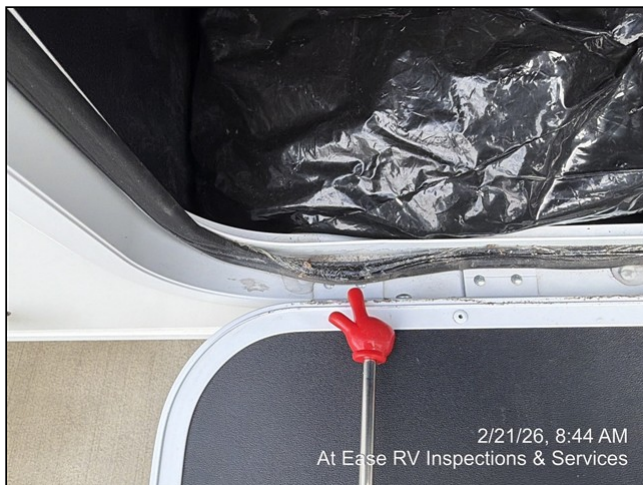
6.4.D Item 1 (Picture) Loose gasket on compartment door
