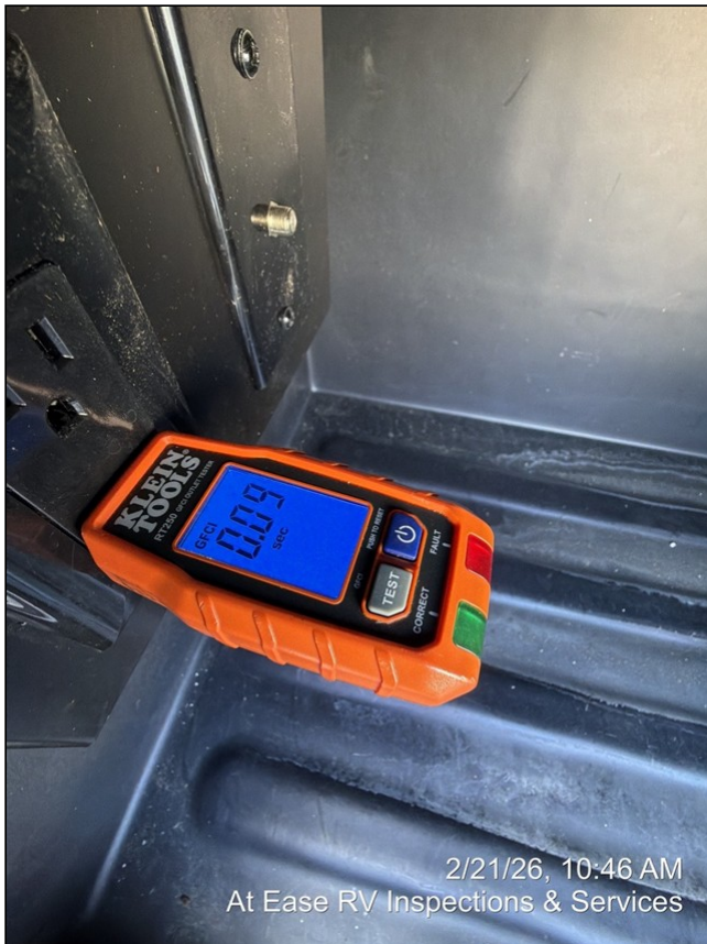
18.12 Item 1 (Picture) GFCI testing
