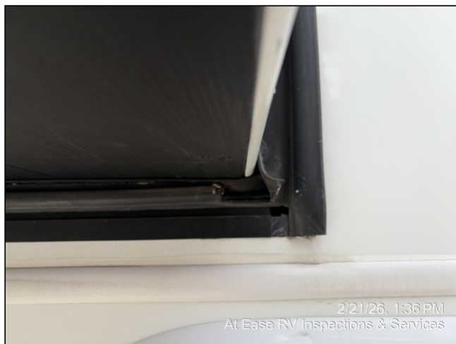
12.6.B Item 1 (Picture) Bottom back corner of slideout sweep
