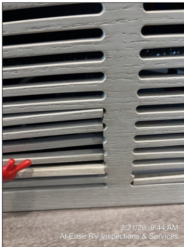
24.24 Item 2 (Picture) Converter/inverter access panel
