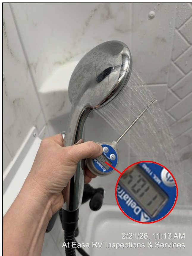
23.14 Item 1 (Picture) Hot water temp on gas
